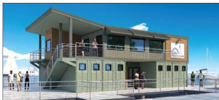
The unique two-story boater amenities building has been constructed from single-use shipping containers, resulting in a modern facility with a retro look.
