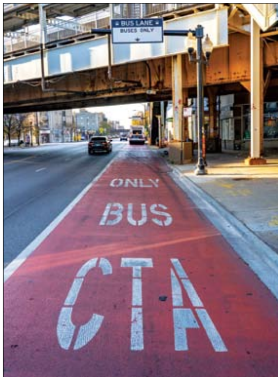
Last week the Chicago Dept. of Transportation began installing red bus-only lanes on Chicago Ave. between Sangamon and Larrabee streets.
