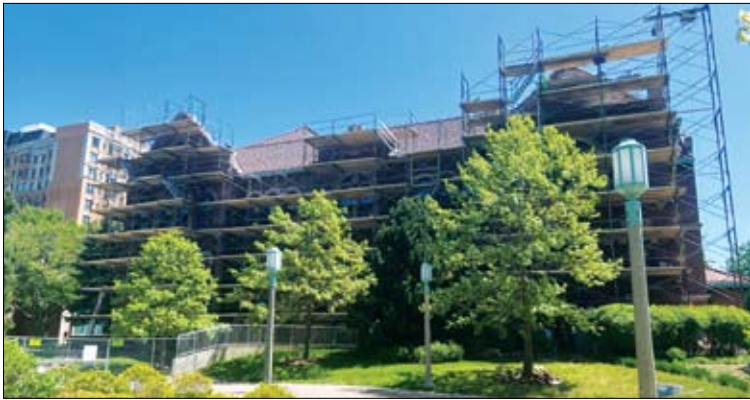
Loyola University's Dumbach Hall facade restoration
