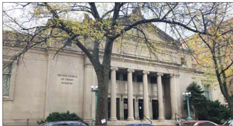
Located at 2700-2717 N. Pine Grove Ave., a developer will incorporate the south, east and west facades of the existing 2nd Church of Christ Christian Science building into what will become a six-story residential building with 22 residential units.
