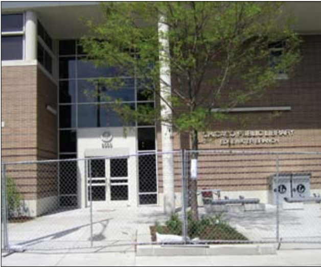
The New Edgewater Library awaits its grand opening at 6000 N. Broadway. Some interior work was still being completed this week.
