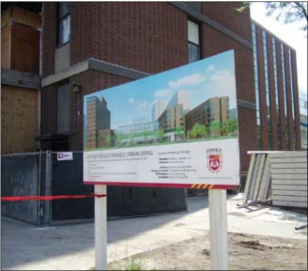
Construction continues on Loyola's Lake Shore Campus Center for Sustainable Living and San Francisco Residence Hall.
