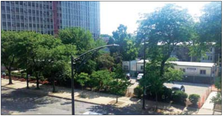
The apartment complex is currently undergoing a complete life safety and modernization renovation. Photo by the 49th Ward office
