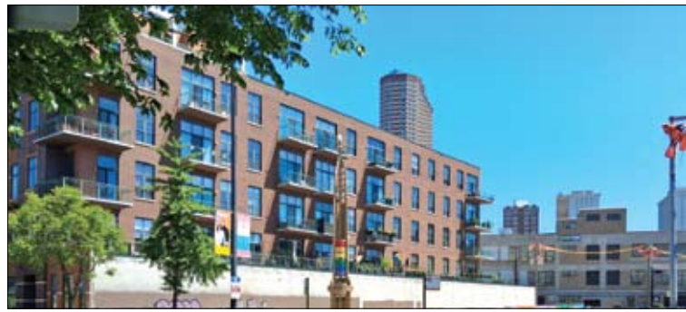
Cordoned-off vacant lot at 3611 N. Halsted St. Photo by Bob Zuley
