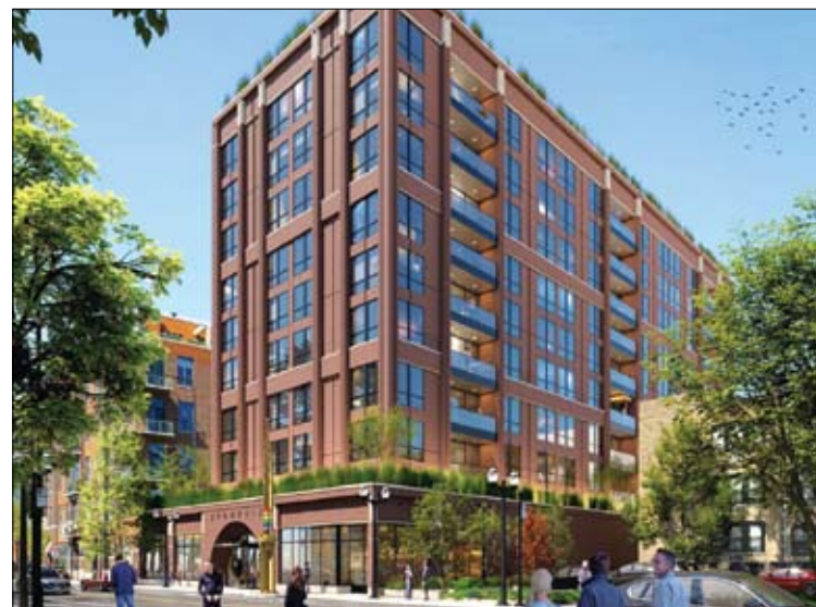
The Phoenix, a 12-story tower planned for 3611 N. Halsted St.
