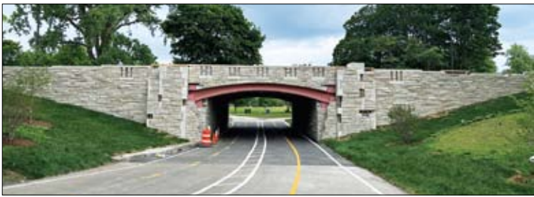
Along with the bridge repairs, the city has wrapped up final paving and drainage work on two Simmonds Dr. underpasses.
