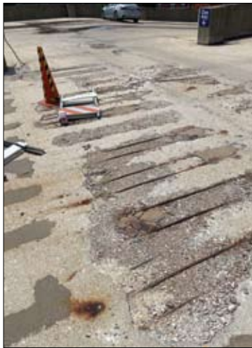
There appears to be a tremendous amount of structural deterioration at Piper's Alley including spalling concrete and exposed reinforcing steel bars on the top floor garage deck.
