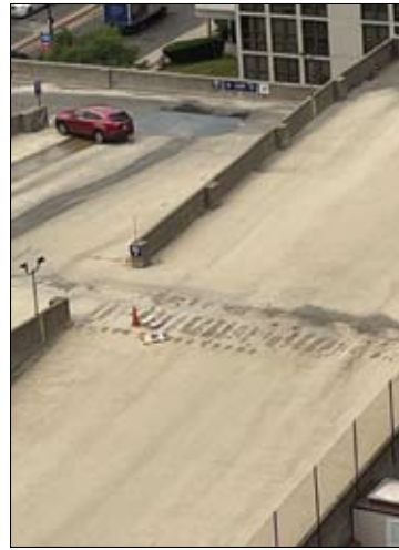
There appears to be a tremendous amount of structural deterioration at Piper's Alley including spalling concrete and exposed reinforcing steel bars on the top floor garage deck.
