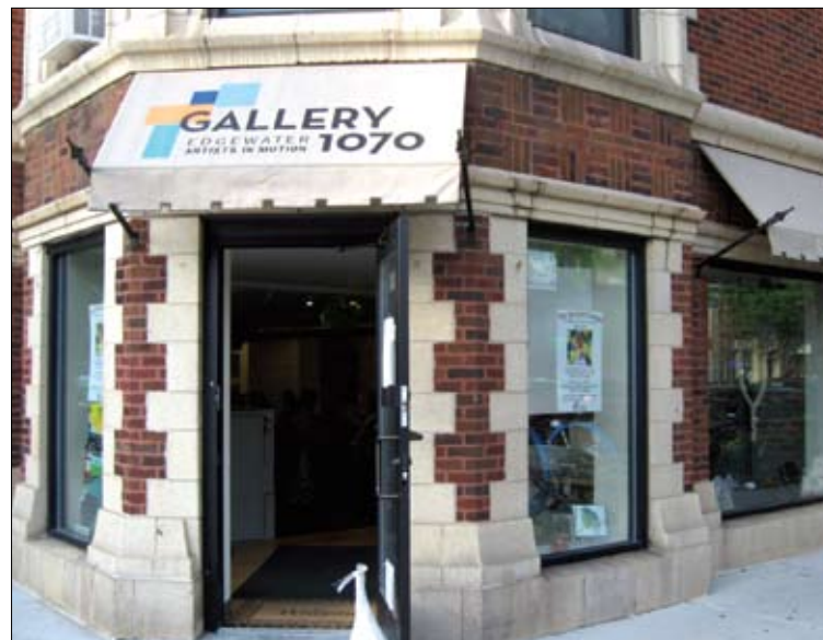
Gallery 1070 on the corner Granville and Winthrop is part of a renovated building that was vacant for over 20 years. The two spaces are now available for exhibits as well as art workshops, private parties and community use.
