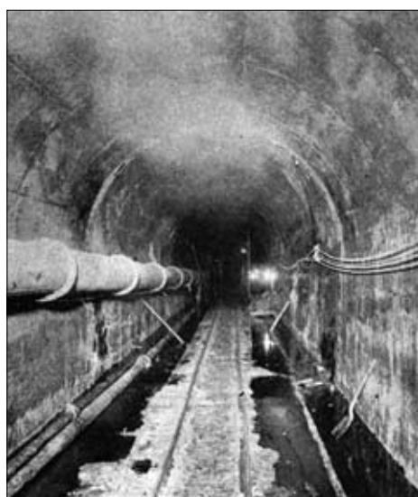
This 1916 photograph shows the interior of one of the water tunnels after completion.
