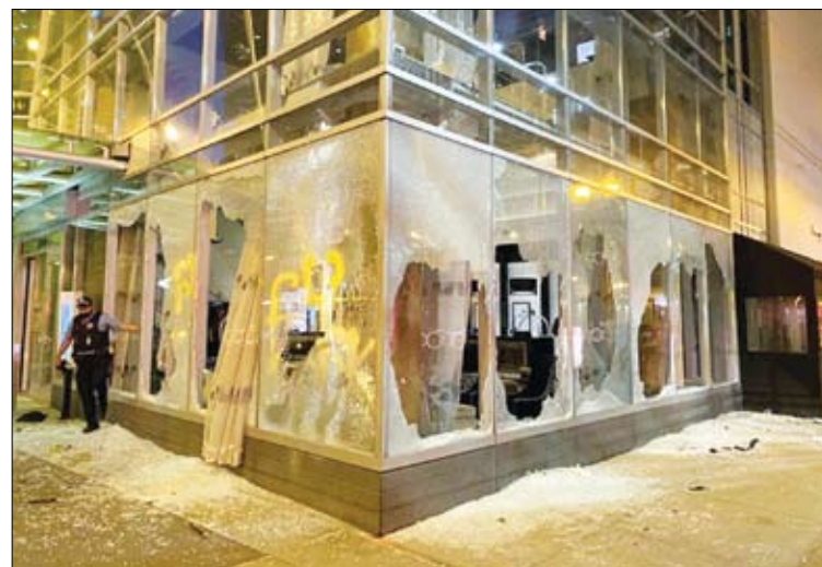
Riot damage to the Wit Hotel at State and Lake streets in the Loop. Photo courtesy of Chicago Loop Alliance
