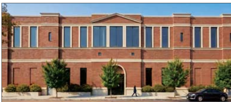
Rendering of the proposed ComEd substation in Lincoln Park at 1111 W. Diversey Pkwy. Courtesy ComEd
