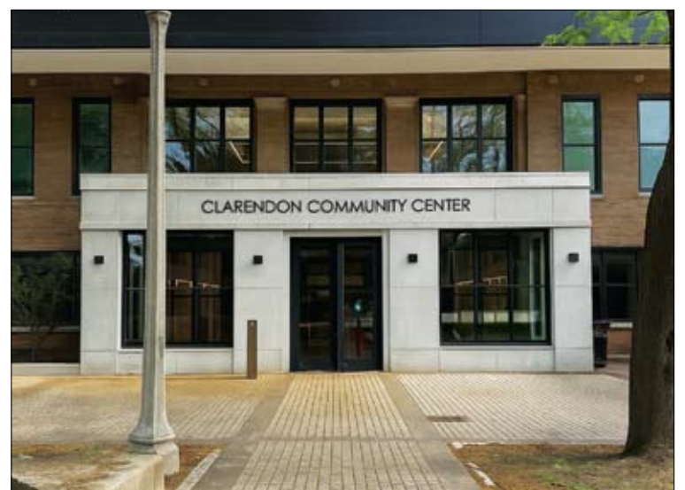
A former Chicago Park District beach house found new life as a field house in Clarendon Park after losing its beachfront location. After $13 million in repairs, it will reopen this weekend. Image courtesy Katharine Boyda, Clarendon Park Advisory Council President
