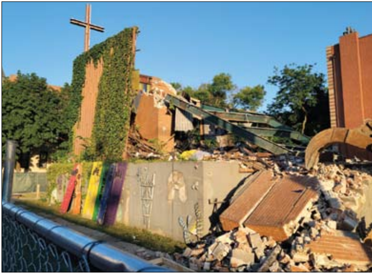
The former Lakeview Lutheran Church at 835 W. Addison St.
