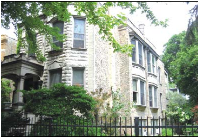
The greystone at 1436 W. Berwyn was built in 1908 by two local Swedish immigrant brothers, Christ and John Christiansen. A development corporation wants to demolish or partially demolish the building to build a four-level building that would include six condos. An online petition was signed by close to 600 residents opposing the project.
