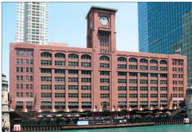
The Reid Murdoch Building, 320 N. Clark St.
