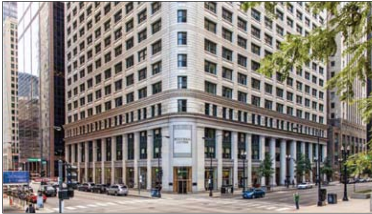
Chicago-based Golub & Company, are reportedly set to surrender the historic 21-story Burnham Center, 111 W. Washington St., in a bank foreclosure.
