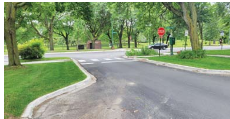
This photo of the 6800 block of N. Bell Ave. shows a new CDOT design that impedes ADA access. The bump outs intentionally narrow the roadway, leaving paratransit drivers facing head on traffic troubles when their vehicles block roadways as they stop to pick up disabled riders. The narrowest, most constricted part of the newly redesigned intersection is where ADA sidewalk ramps meet the roadway, removing any buffer between the disabled and their mode of transportation, and oncoming traffic.
