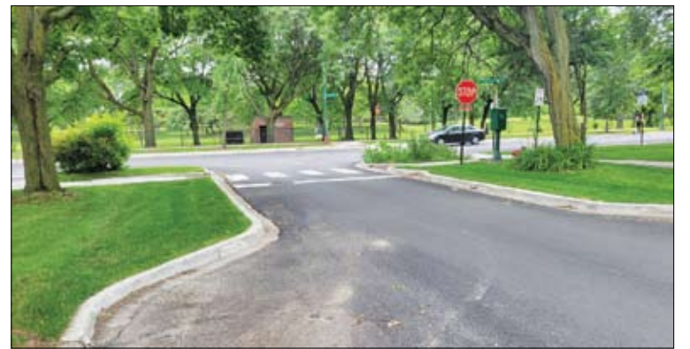
This photo of the 6800 block of N. Bell Ave. shows a new CDOT design that impedes ADA access. The bump outs intentionally narrow the roadway, leaving paratransit drivers facing head on traffic troubles when their vehicles block roadways as they stop to pick up disabled riders. The narrowest, most constricted part of the newly redesigned intersection is where ADA sidewalk ramps meet the roadway, removing any buffer between the disabled and their mode of transportation, and oncoming traffic.
