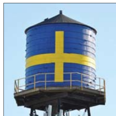
A replica of the original water tank is being assembled in the parking lot and will be installed soon on the Swedish American Museum's rooftop.
