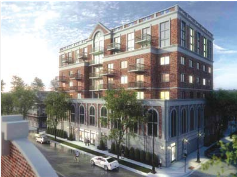
Ald. Joe Moore [49th] has agreed to support the construction of a proposed new eight-story building at 1313 W. Morse.
