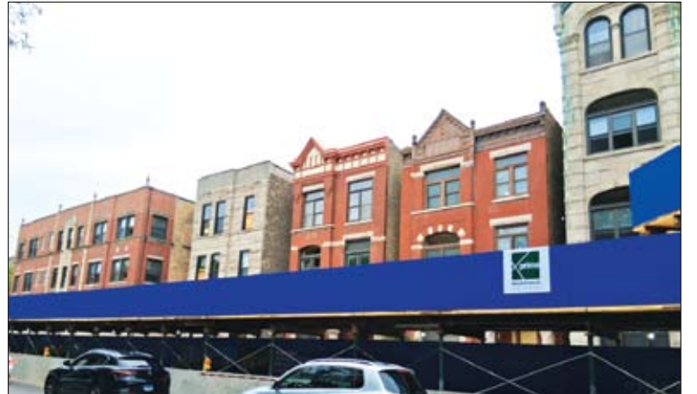
Demolition has begun on five vintage buildings on the 2300 block of N. Sheffield Ave. Photo by Bob Zuley
