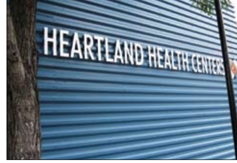
The new Heartland Health Center at 1300 W. Devon was the site for the July 28 community meeting.
