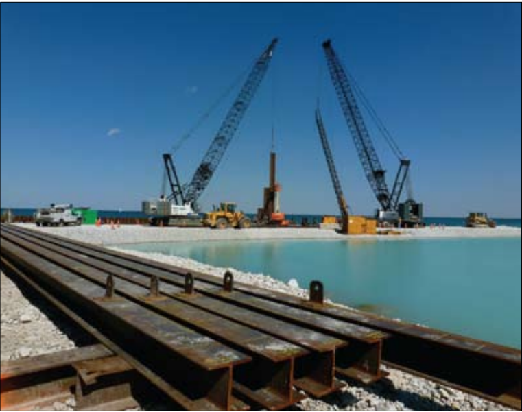
Giant steel poles, or pilings, are pounded 80 feet into the sand and then attached at the visible eyelet to the horizontal sheeting for lateral stability.
