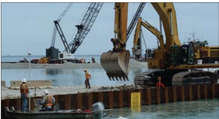
The south end of the project where stone is being shoveled in front of the sheeting to act as a wave breaker and to prevent erosion.
