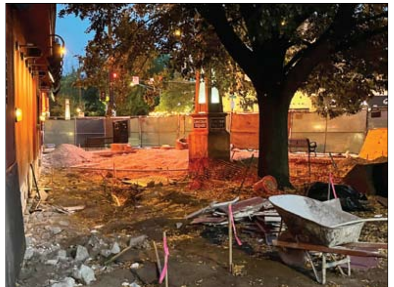
The new outdoor patio under construction at Lincoln and Montrose avenues.
