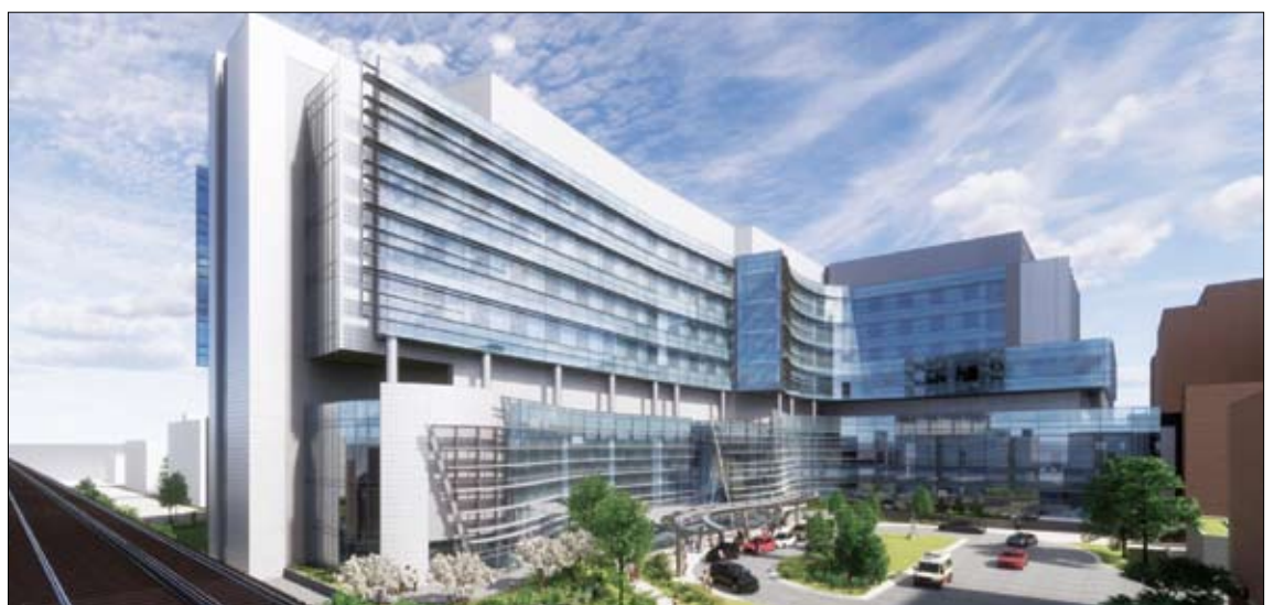
Work is progressing on a massive new $645 million expansion at Advocate Illinois Masonic Medical Center in Lake View.
