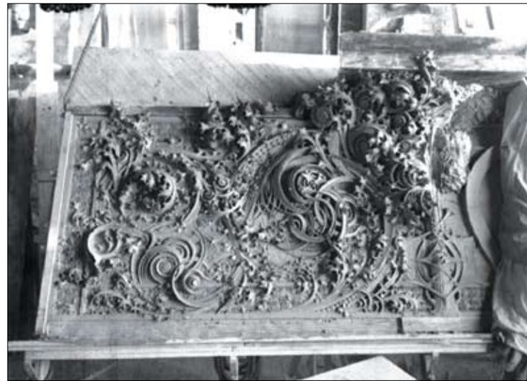
Found tucked in an old storage facility at the Univ. of Wisconsin-Milwaukee are original molds for the ornamental terra cotta used in the construction of the 1 S. State St. building. These molds were rescued by a professor from the Architecture Dept. They were about to be thrown away when it came time to clear out the building.
