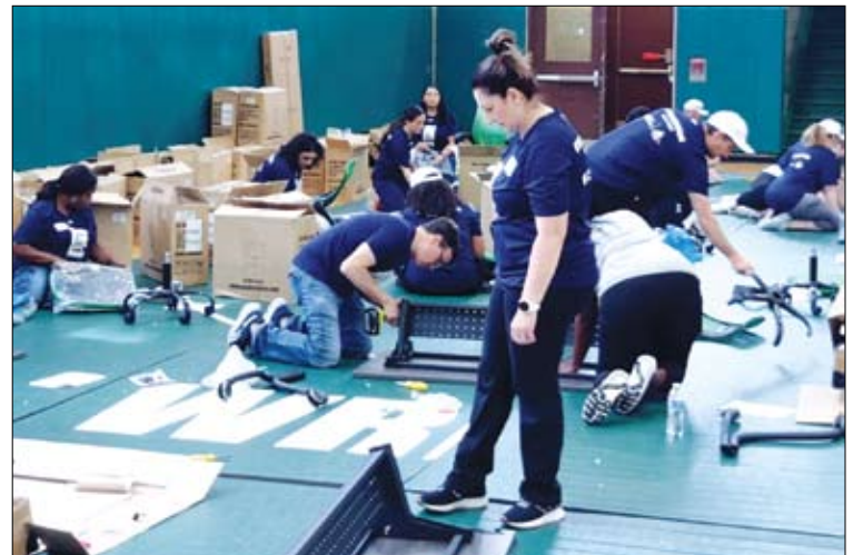
Volunteers prepare a floor area for a new surface in the weight room at Senn High School, 5900 N. Glenwood in Edgewater, as part of the Cal Ripken, Sr. Foundation’s 2023 Team8Tour. Photo by Joanne Kitsos
