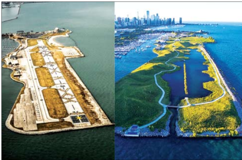
Meigs Airport (left) before it was demolished in the dead of night. Northerly Island (right).
