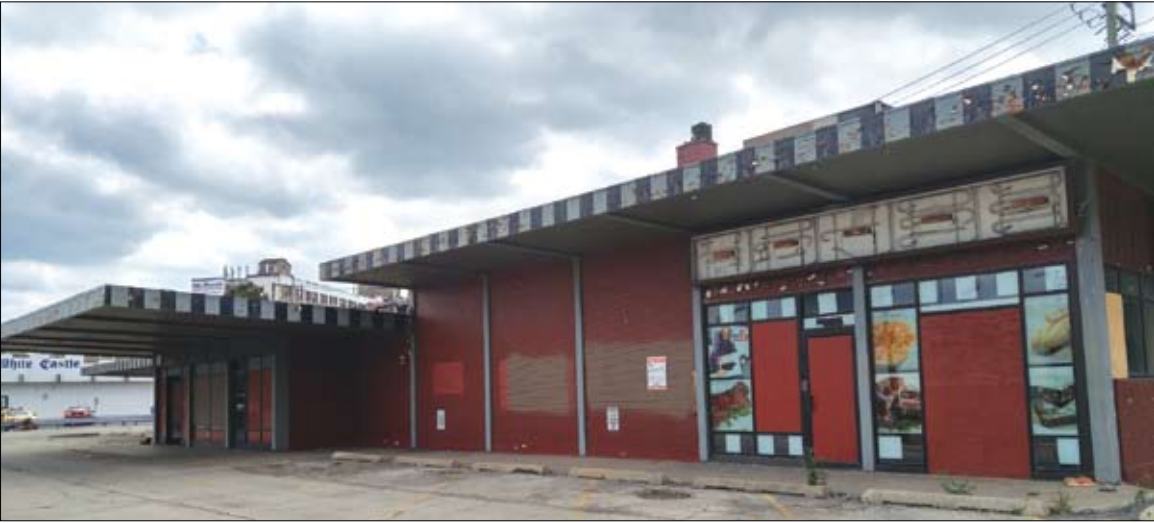
The eyesore formerly known as Carson's Ribs, 5970 N. Ridge Ave. is expected to be demolished, rebuilt and serving Starbucks coffee by mid-2018.
