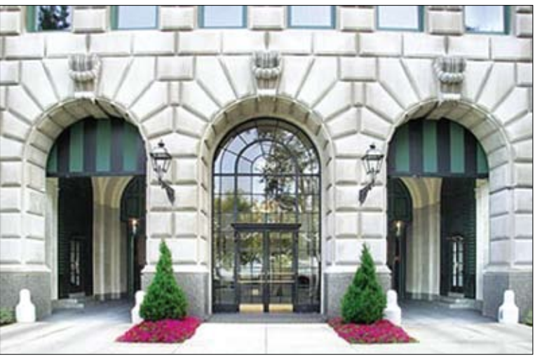
209 East Lake Shore Dr., an 18-story luxury co-op in the Gold Coast, sued on May 14 for violation of the city's new Life Safety ordinance. The housing complaint was dismissed on Aug. 5 with only one court appearance.
