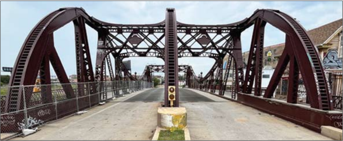
When the Cortland Street Bridge closed in 2025, the bridge had been scheduled to have its bridge deck, steel floor system, and counterweights repaired, and install new concrete-filled grating, timber sidewalks, railings, and lighting replaced. Now the bridge may have to be completely rebuilt.
