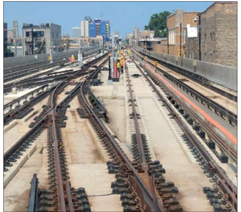
A view north up the Red Line tracks.
