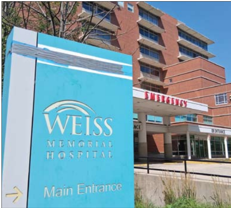
Weiss Hospital sign with duct tape newly covering Emergency.
