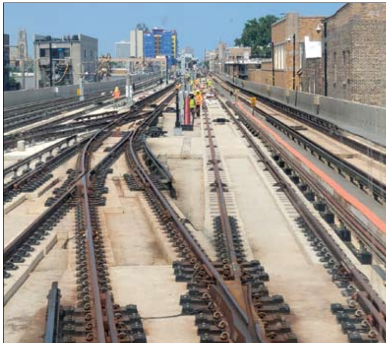
A view north up the Red Line tracks.
