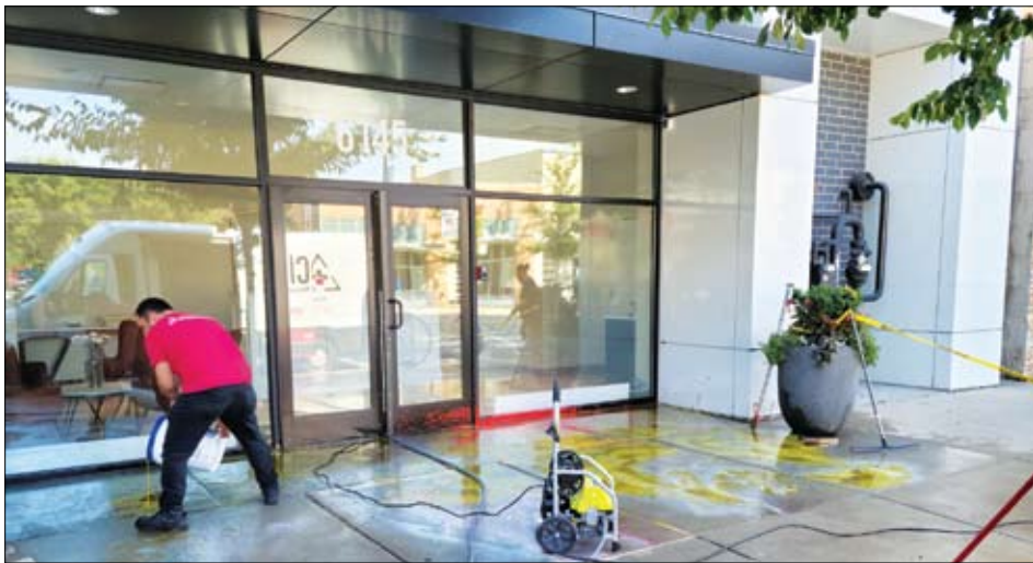
Worker cleans up vandalism at 6145 N. Broadway.
