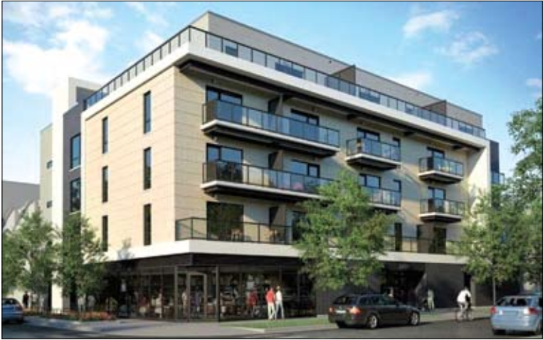
The new TOD project that is just getting underway at 4618-4620 N. Western Ave.
