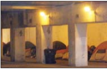
The "tent city" under the Wilson Ave. viaduct.
