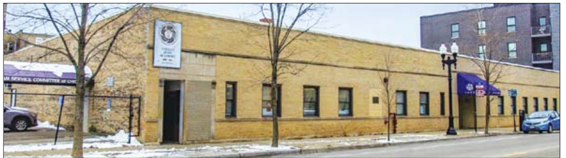
Despite the heavy equipment on the block, the Japanese American Service Committee, 4427 N. Clark St., says they are not yet vacating their property for a demolition. The social service organization will at some point in the future move to the 5700 Block of Lincoln Ave., and Black Ensemble Theater will take over their former Clark St. property. Photo courtesy Uptown Update
