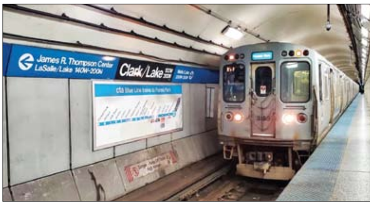
A train arrives at the Clark-Lake Blue Line station below the James R. Thompson Center, now Google.
