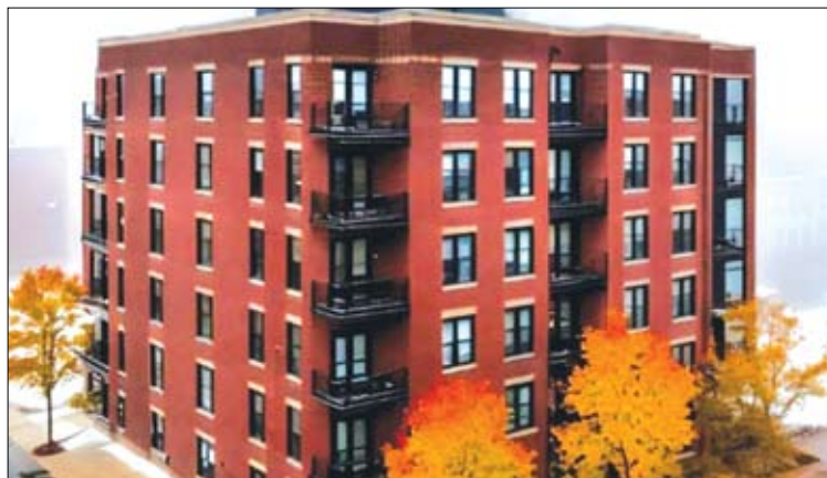
Prior to the onslaught of Transit Oriented Developments, a project such as the one at 5054-56 N. Ashland would have required the developer to include 32 off-street parking spots for future tenants.
