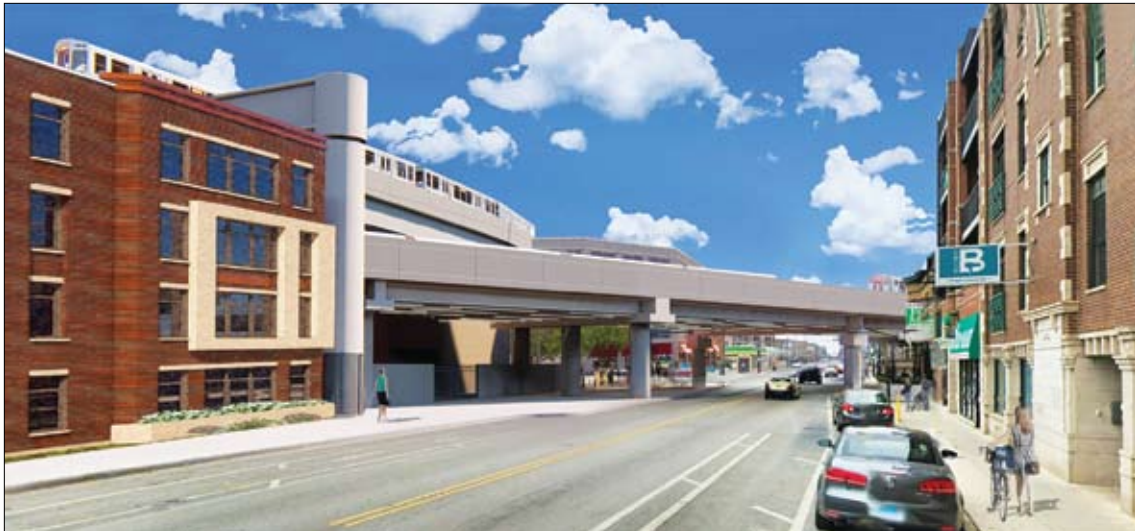
This is what the Clark Junction is projected to look like. It is the point where the Brown Line tracks will 'fly over' the Red and Purple lines, meeting up again just north of the Belmont CTA station.
