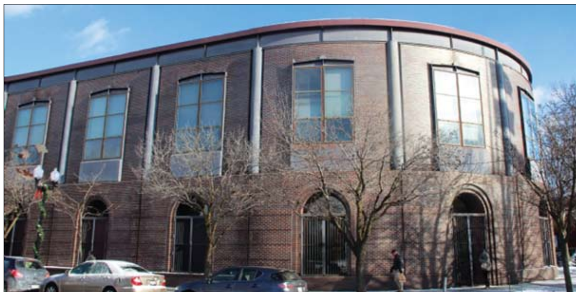
The Sulzer Library will be closed for repairs from Oct. 16 through Nov. 5, but you'll still have to return your books on time.
