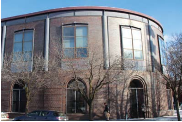
The Sulzer Library will be closed for repairs from Oct. 16 through Nov. 5, but you'll still have to return your books on time.
