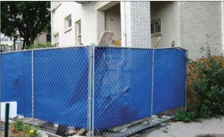
Renovation work includes rehabbing the rear entrance as well as the south mansion at 6205 N. Sheridan. An open house will be held Oct. 17
