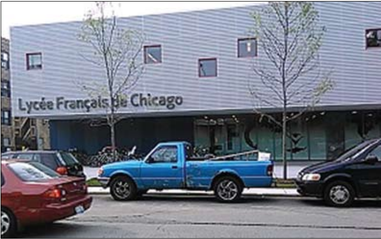
On Sept. 1, the Lycée Français de Chicago officially opened its new $35 million, 3.8-acre Spanish-and-American-designed campus in the city's Ravenswood area.
