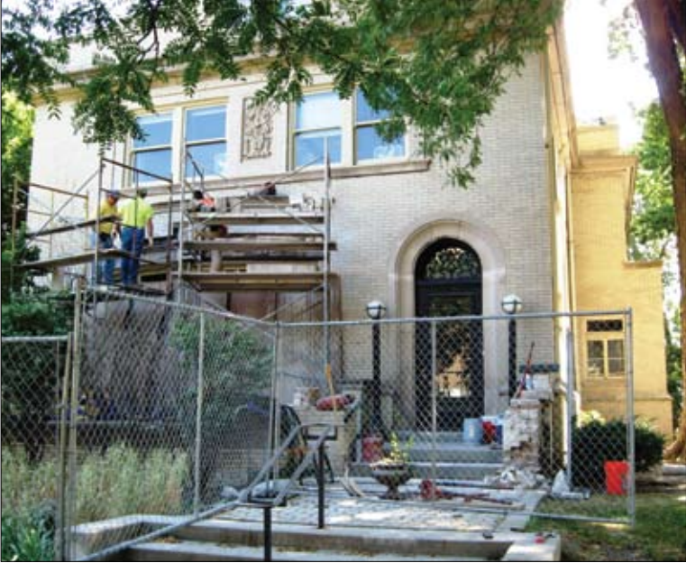
Workers address façade issues at Gunder House (North Lakeside Cultural Center) at Berger Park. The Chicago Park District purchased the house in 1981 and will rent out six rooms and use other space for arts partners.
