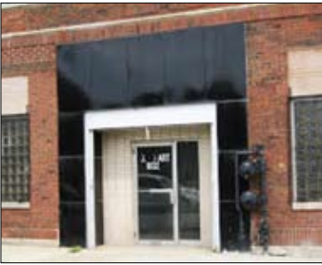
The former 35,600-square foot Duro Art building at 1832 W. Juneway Ter. will be demolished.
