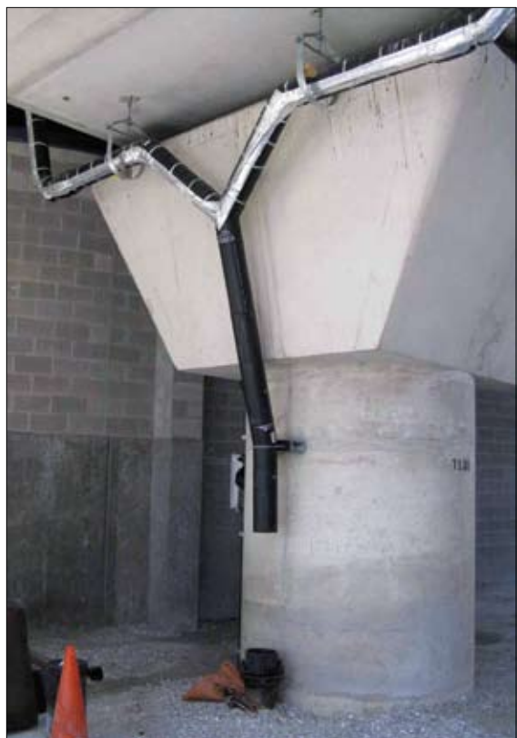
The downspout gutters (left) leading from the Red Line end four feet above the ground and may be responsible for flooding that closed the Baton Show Lounge in Uptown, whose back door (right) was adjacent to the gutter.
