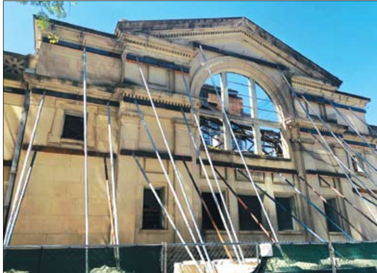
Work has begun in Lincoln Park as developers begin to insert a huge six story building into the middle of what once was The Second Church of Christ Scientist. Already gone to dust and sky, (as is evident in this photo) is the beautiful domed ceiling that was once the architectural centerpiece of this 120 year old Church. Photo by Jim Matusik
