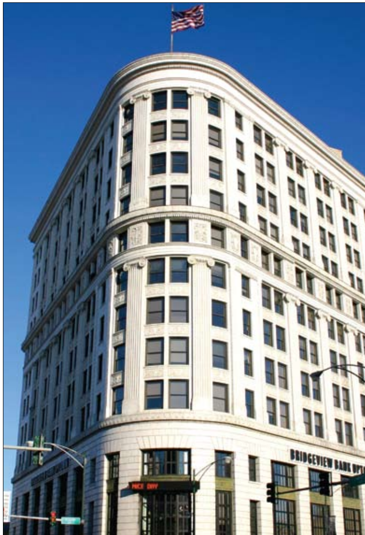
For 39 years, the historic bank building at 4753 N. Broadway Ave. has been home to RefugeeOne. Photo by Sheila Swann
