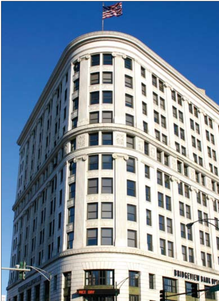
For 39 years, the historic bank building at 4753 N. Broadway Ave. has been home to RefugeeOne. Photo by Sheila Swann
