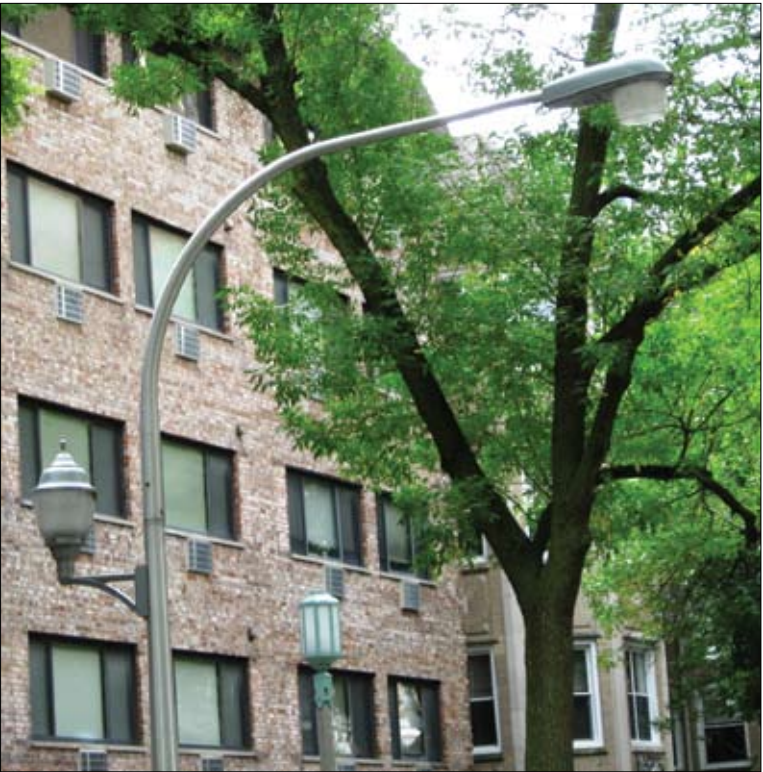
Installation of the acorn-style streetlights will begin on four streets in the 49th Ward this week.
