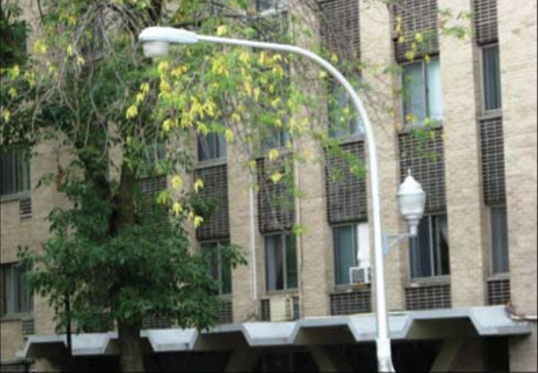
The new acorn-style streetlights feature a second light that illuminates the sidewalk, thus enhancing pedestrian safety.
